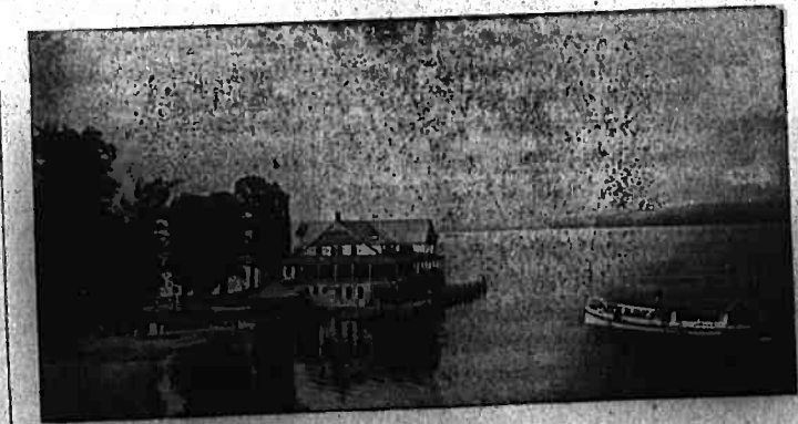
Old Pier Building, erected in 1886, to be torn down at the end of this year.
